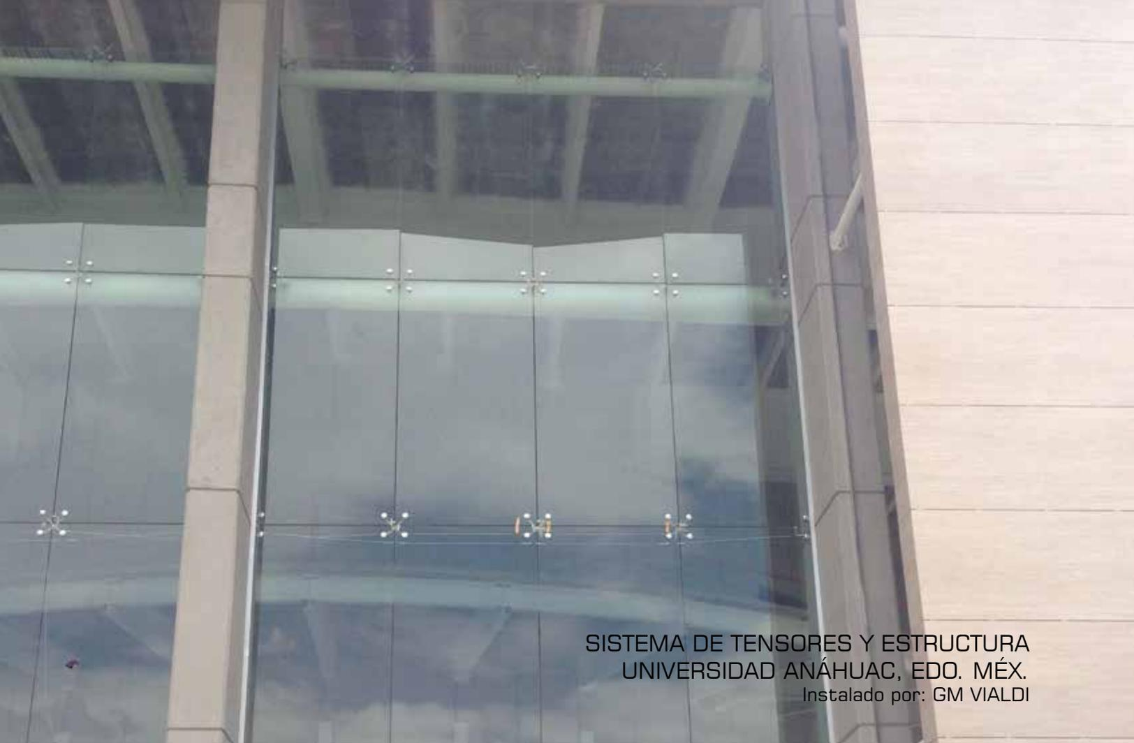
SISTEMA DE TENSORES Y ESTRUCTURA
